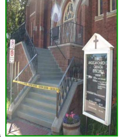
hired to stop water leaks from the front stairs but the client only had a 1-day window to complete this project. Vector Construction decided to apply Advanced Polymer Technology Corporation Qualideck system for its nonskid; high chemical, abrasion and impact durability; resistance to thermal shock with excellent crack bridging and waterproofing capabilities. This project was completed on time and on budget.
