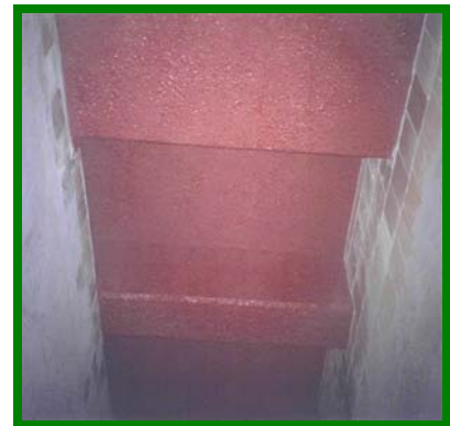
Concrete Ceiling and Beams Coated
