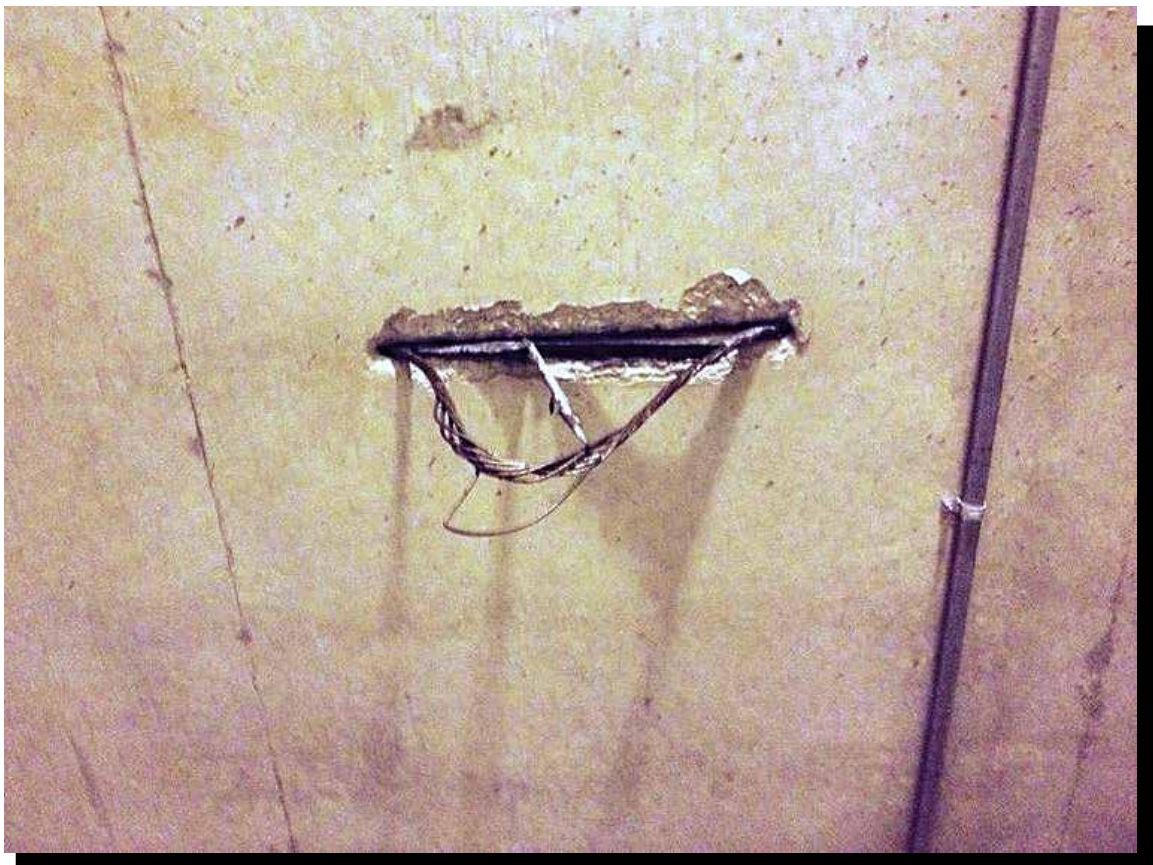
Figure 1: Erupted Post-tensioned Tendon Discovered March, 2013
