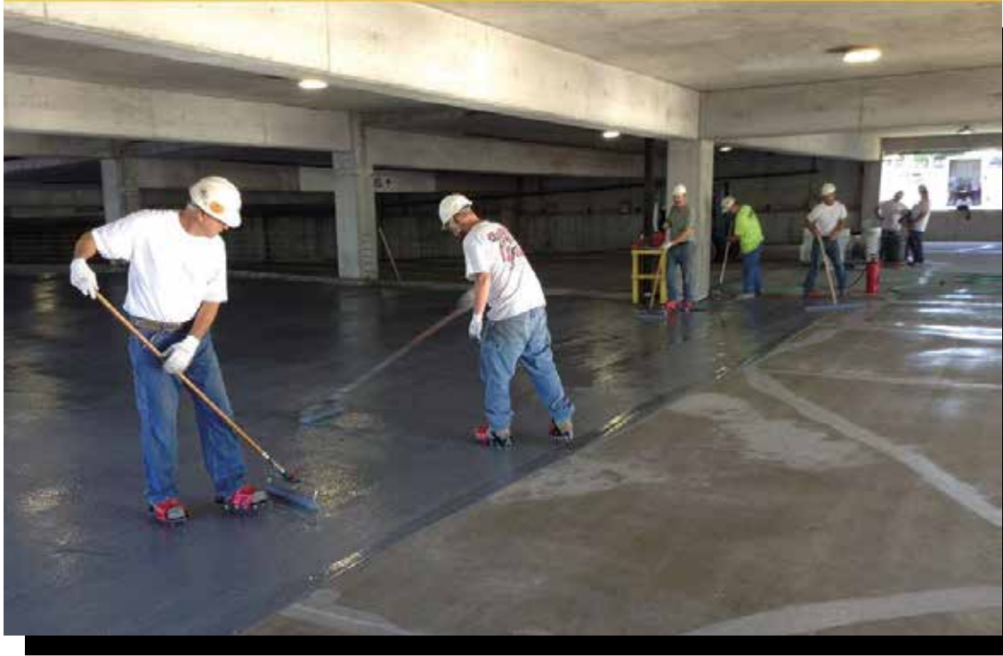
Figure 9: Application of Waterproofing Membranes
