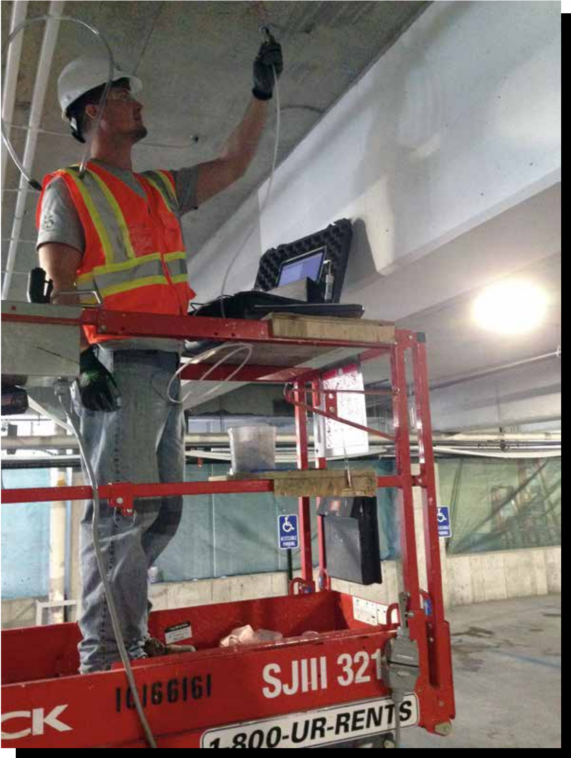
Figure 6: Post-Tensioned Slab Corrosion Evaluation Procedure (moisture test)
