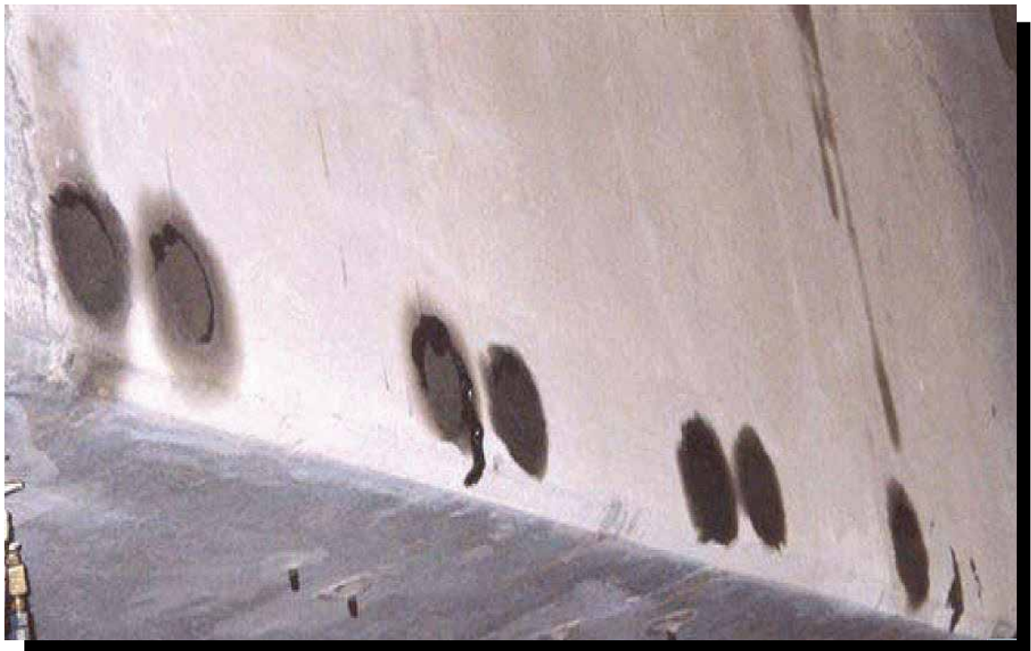
Figure 12: Post-tension Re-Greasing at Grout Pockets
