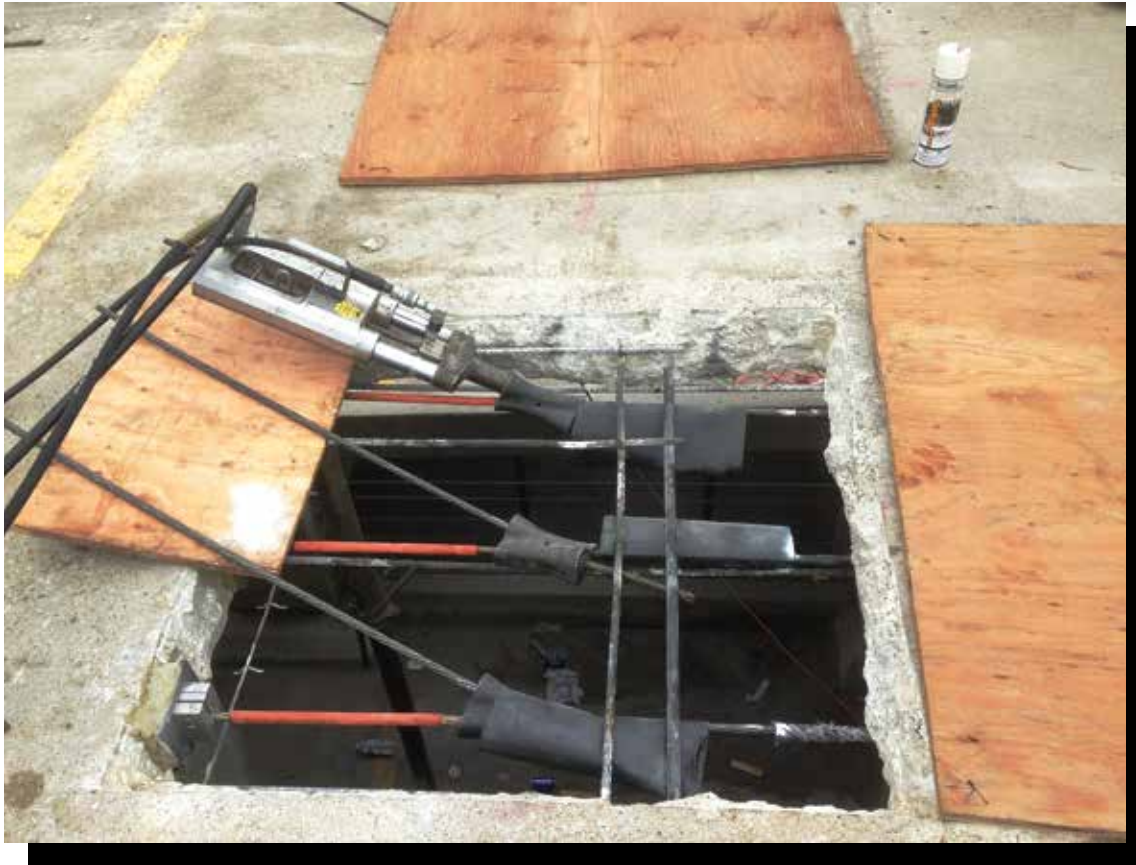
Figure 7: Post-tension Splicing with Center Stressing Chuck
