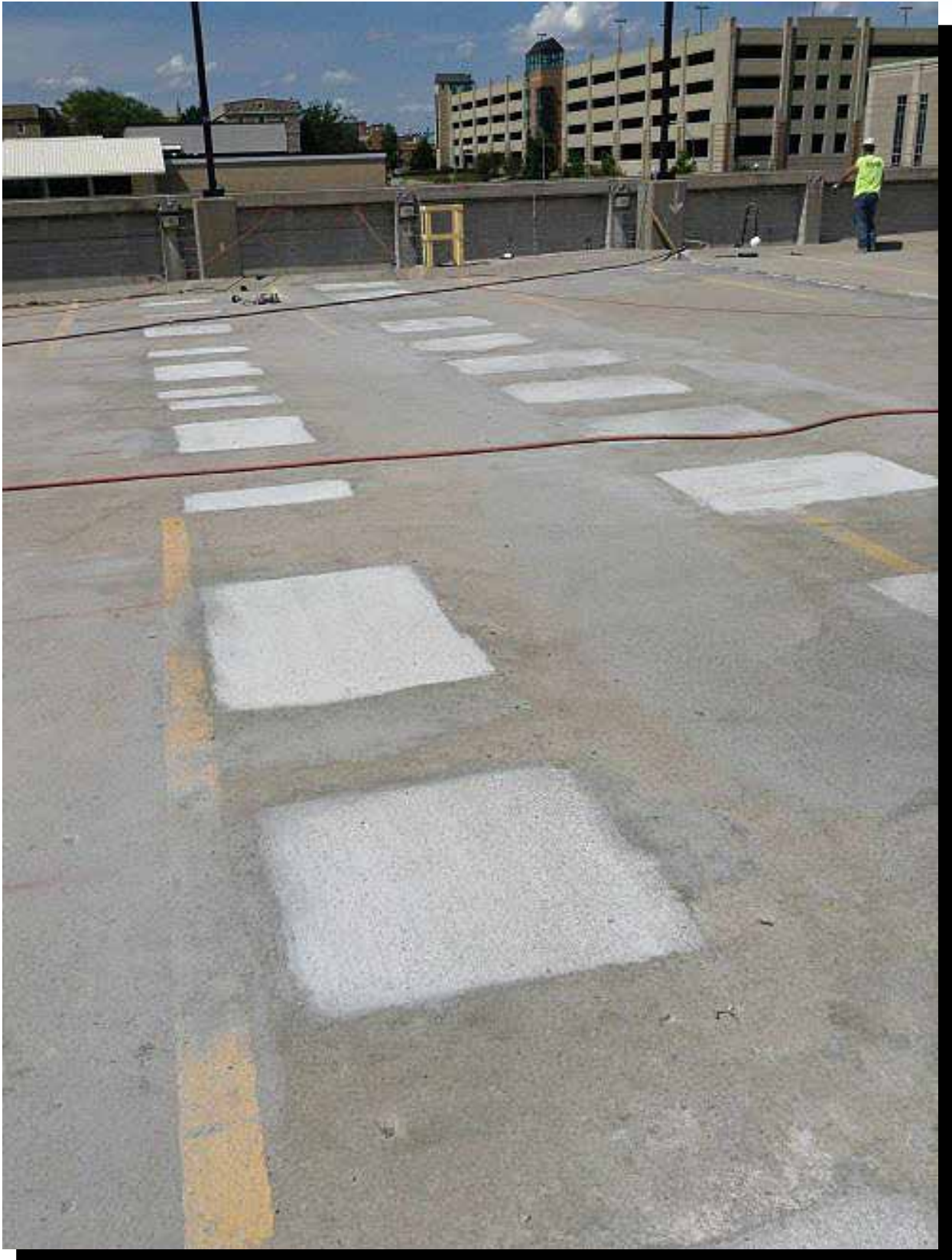
Figure 8: Completed Post-tensioned Slab Repairs
