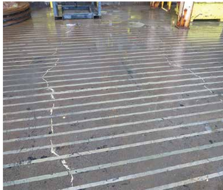
Slab Strengthening and Repairs Completed
