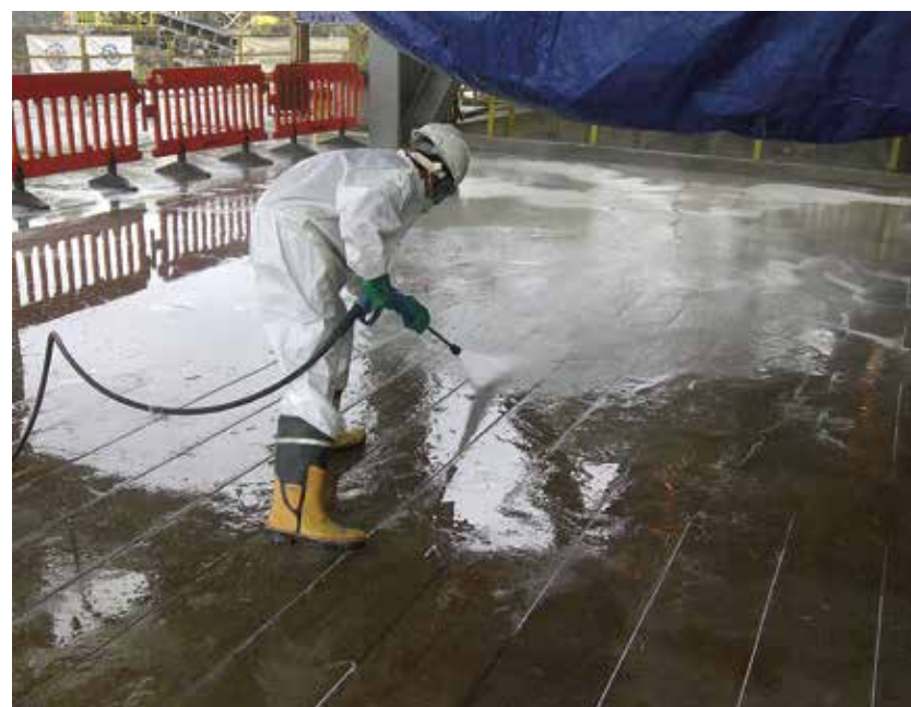
Water Blasting CFRP Slots
