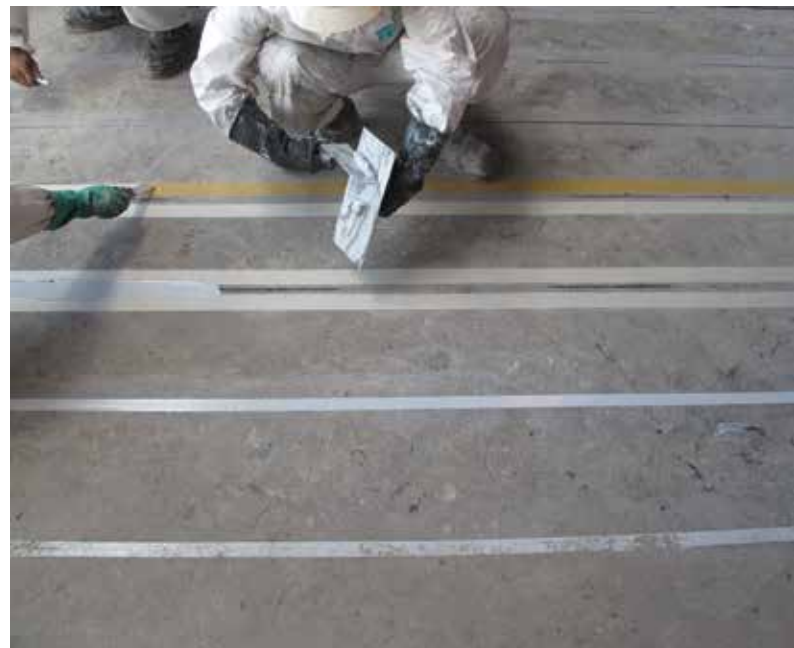
Sealing Top of Slots with Epoxy
