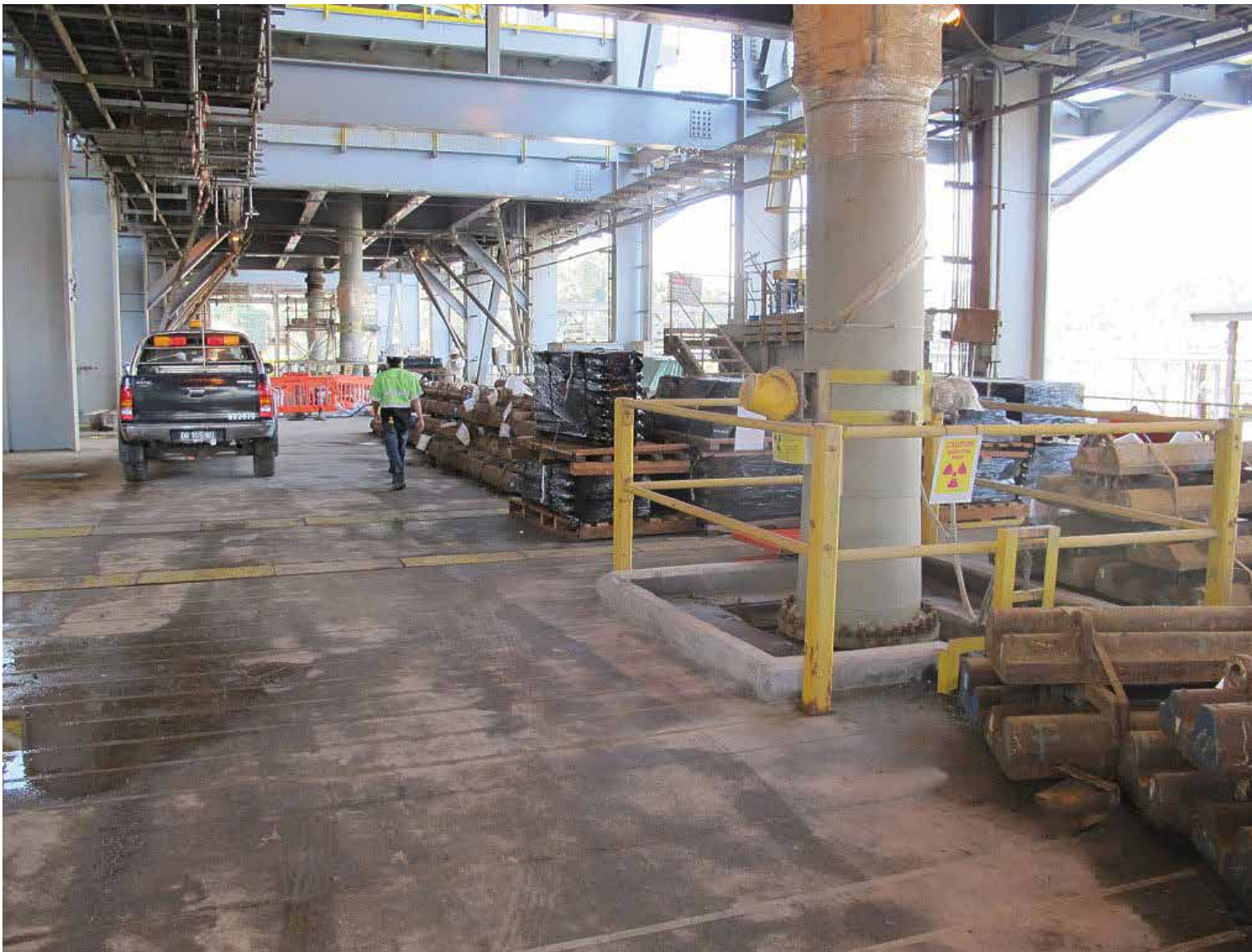
Heavy Steel Mill Liners in Place on Strengthened Floor
