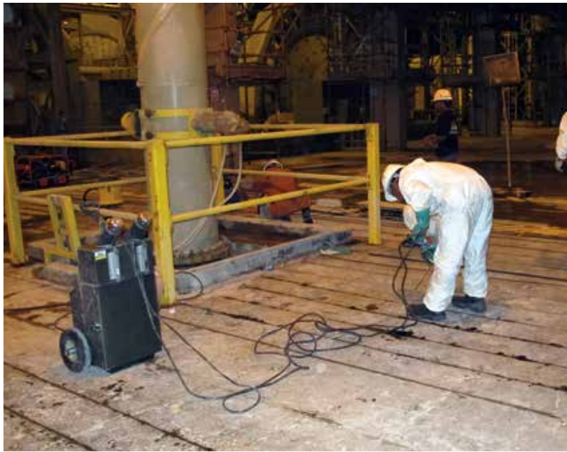
Installing CFRP with Epoxy Injection Pump
