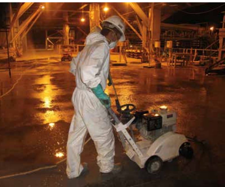
Cutting CFRP Slots
