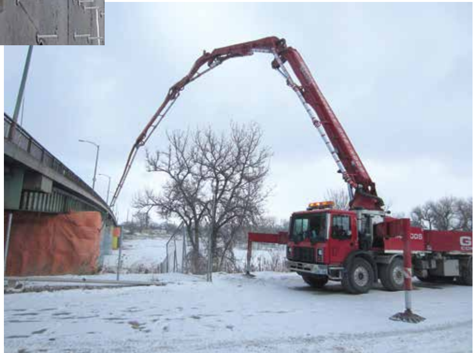
Pump Truck Delivering Concrete for the Repairs
