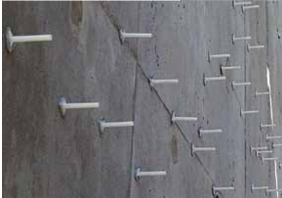
Ports in Place for Epoxy Injection Crack Repair
