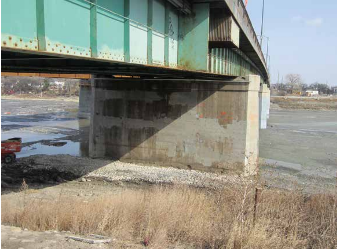
Completed Concrete Repair of Red River Bridge Pier
