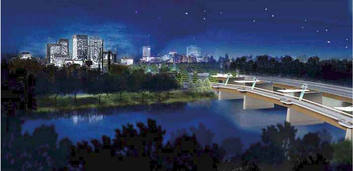
Conceptual Drawing of the Red River Bridges – the Existing Bridge Piers were Rehabilitated and used to Support the Pedestrian Bridge
