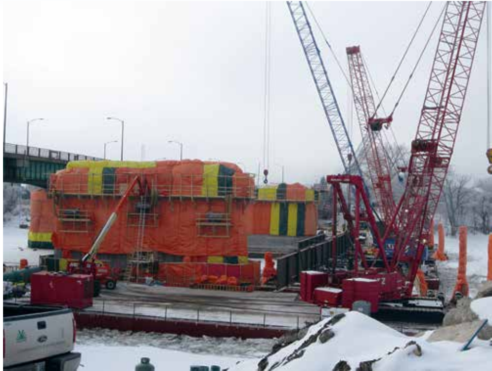
Repair and Corrosion Mitigation of Piers Proceeded inside Heated Enclosures
