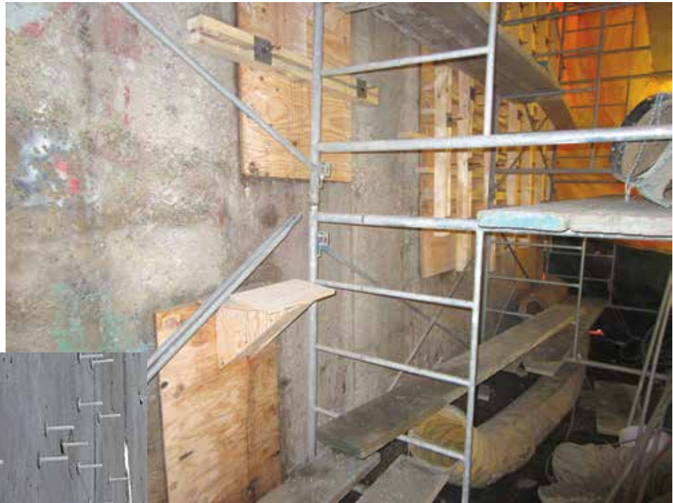
Plywood Formwork in Place
