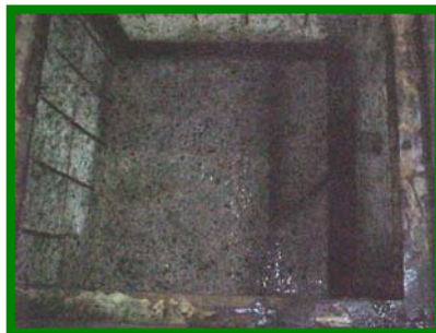
Deteriorated Sump
