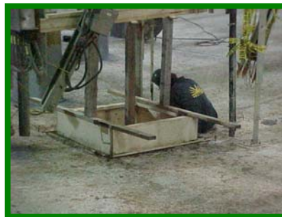
Forming Repair System
