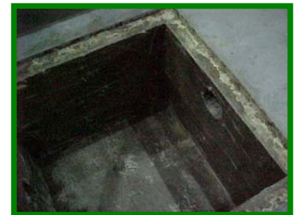
Sikadur EPC Repair Completed
