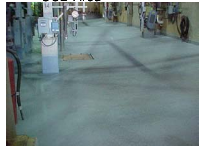
Ucrete HF Installation Completed
