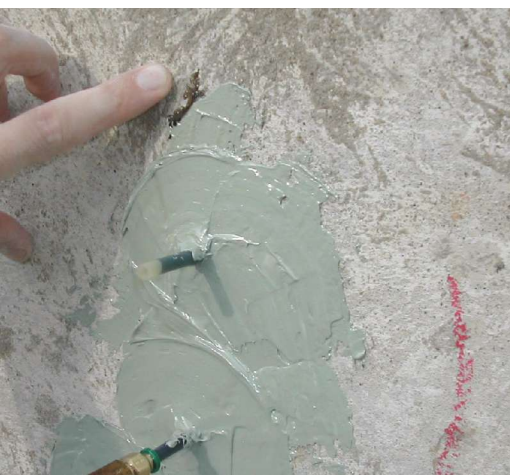
Epoxy emerging from port and hairline crack not previously visible.
